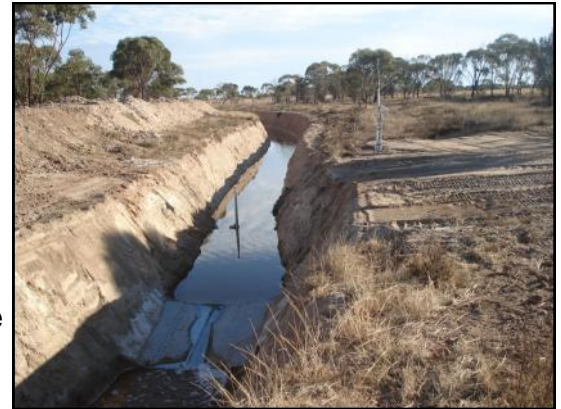
The fully operational crump weir
